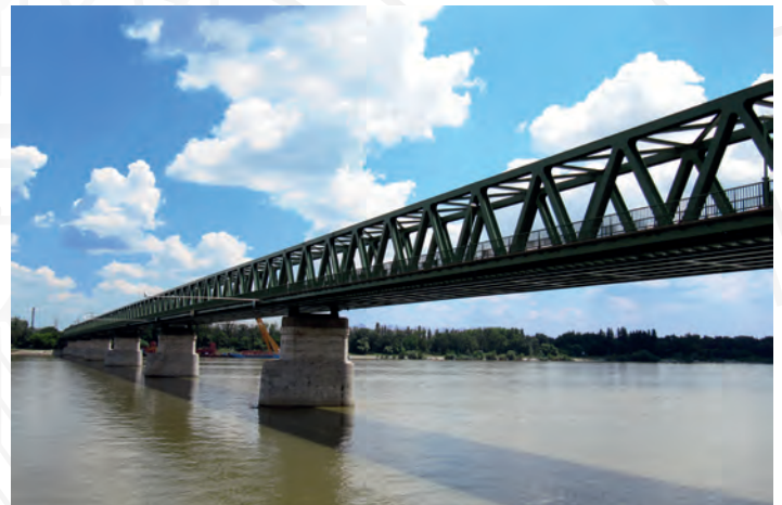
Inspection of Northern Danube rail bridge
