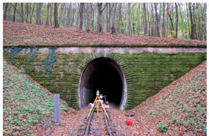
Tunnel inspection of Great Hárs-hill
